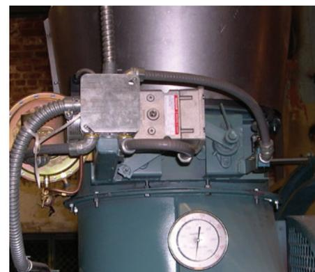
Also, in this case, the auto damper control will regulate the pressure at the vent stub during firing. This will aid in keeping the burner's air/fuel ratio in the proper range at all firing rates.
